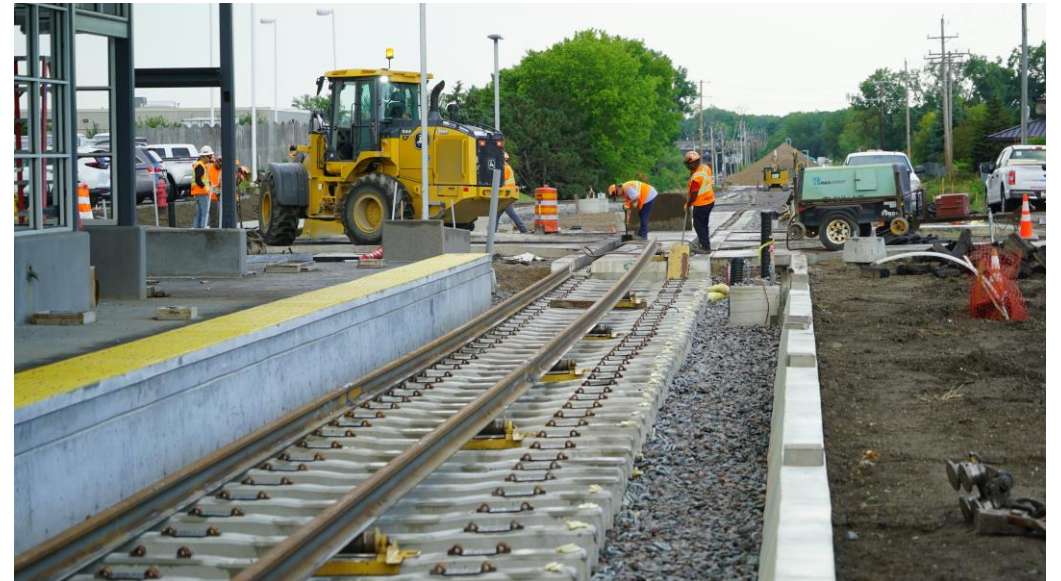
LRT track at the Downtown Hopkins Station
