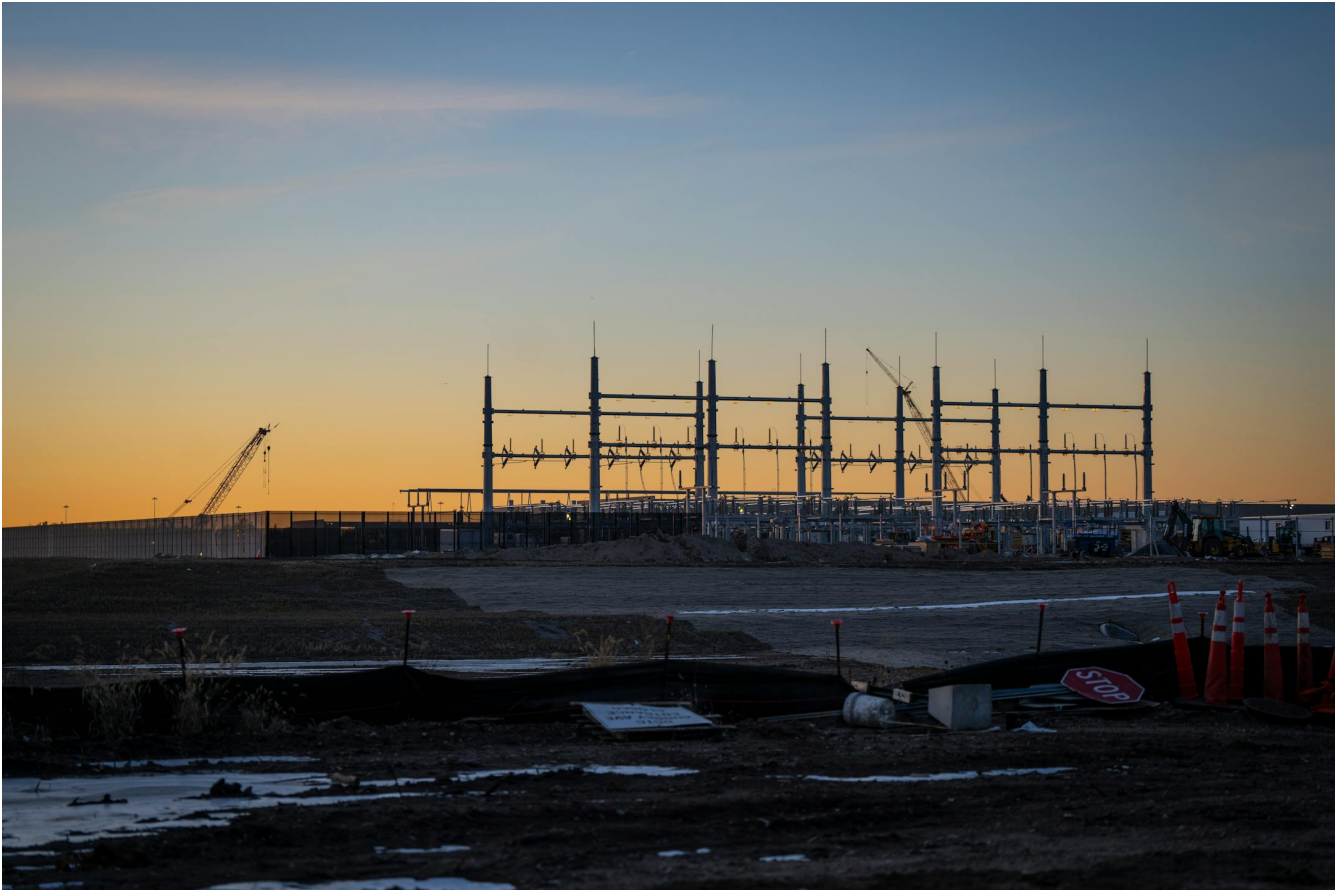
The construction site of the data center in Rosemount on January 7, 2025. (Renée Jones Schneider/The Minnesota Star Tribune)
