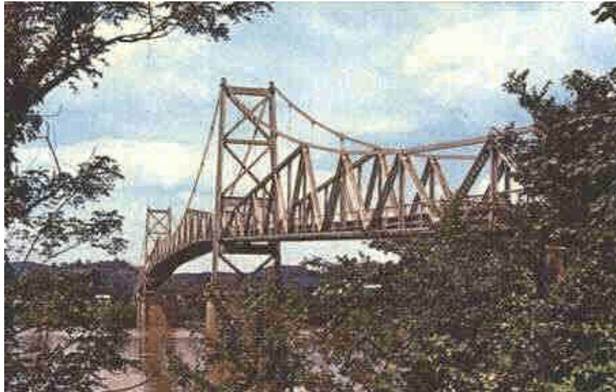
The Silver Bridge , courtesy of Mason County, WV, Web page, Infamous Bridge Disasters (visited Oct. 30, 2007) < http://filebox.vt.edu/users/aschaeff/silver/silver.html >.
